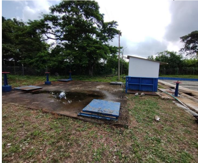
Tanque PTAP Jordán
