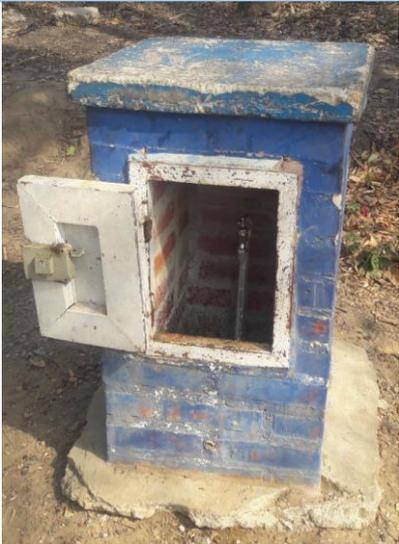
A blue-painted concrete water sampling point with a white door, situated outdoors on a concrete base. |
